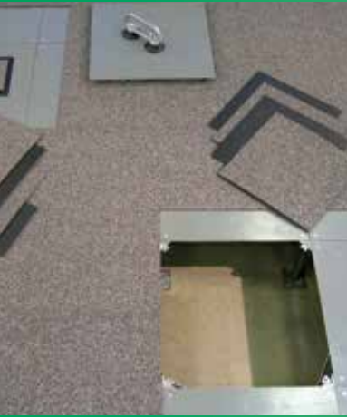
Step 1: Remove four cut carpet tiles from around service box...
