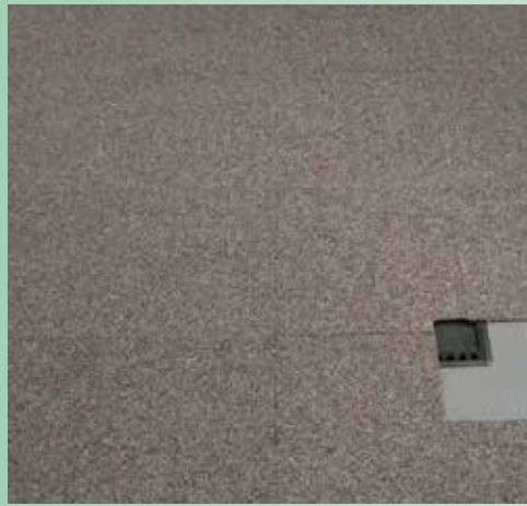
Step 6: Cut carpet tiles do not fit at new location, need new carpet tiles...
