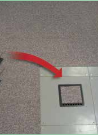
Move cut carpet tiles to service box location...
