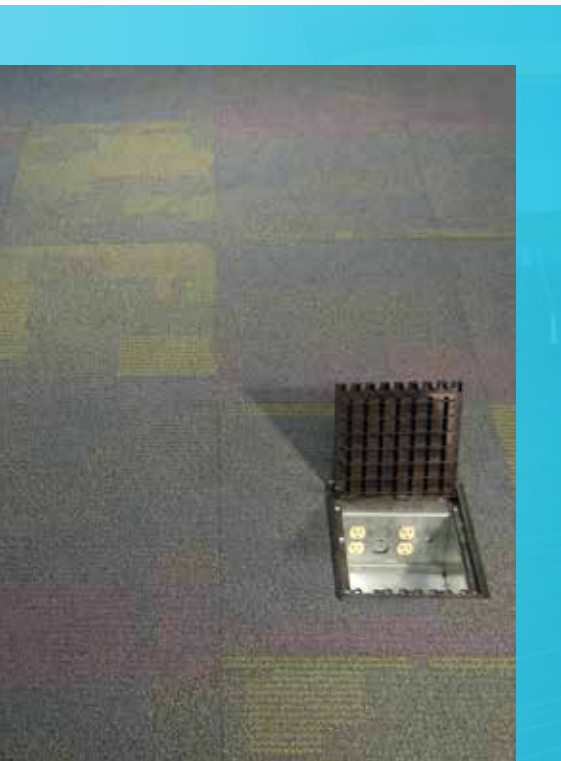
Completed! Process is faster, and waste.
