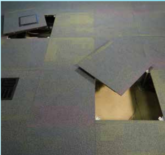
Step 2: Remove access floor panels....
