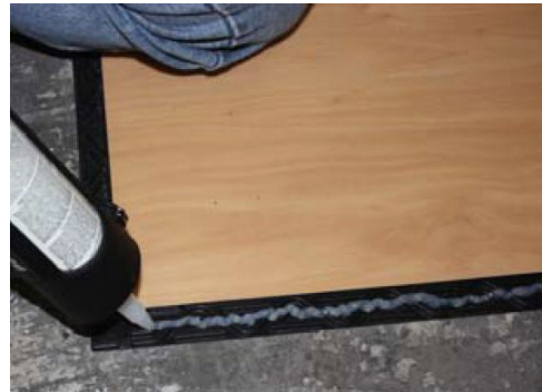
Seam sealer for watertight installation
